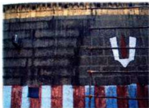
A Part of the Moss and Lichen Affected Wall at Arulmigu Parthasarathy Temple, Chennai after Chemical Cleaning
