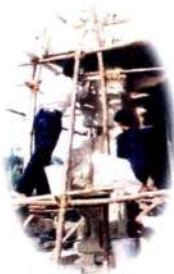
Removing Soluble Salts by Poulticing at Shore Temple, Mahabalipuram
