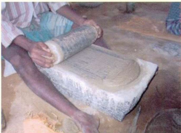
Traditional grinding of lime mortar
