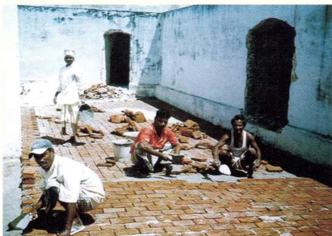
Laying special type of brick floor tiles at Manora
