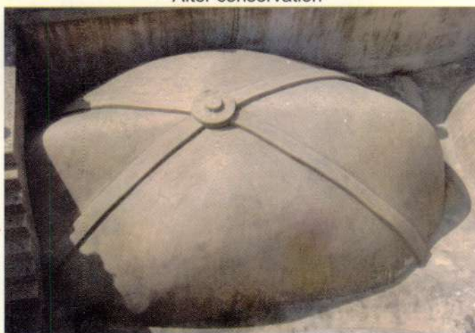
Dansborg - Closeup view showing one of the four domes after conservation - note the central steel cap covered with combination mortar plaster
