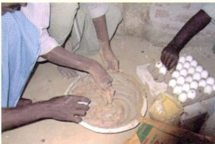
White of eggs used in lime mortar for Moghul plaster
