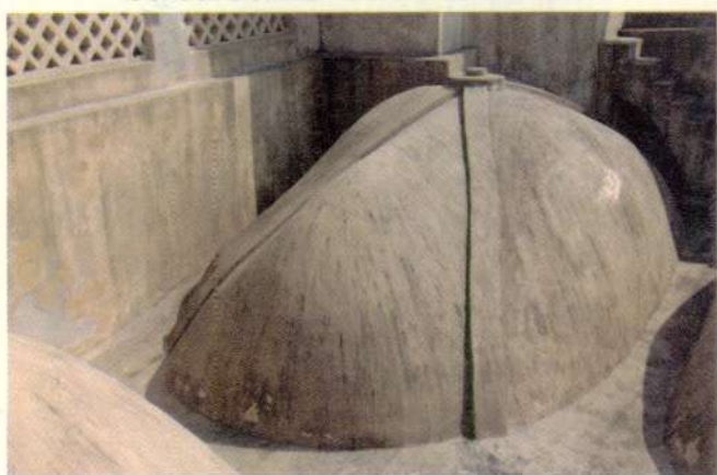
Dansborg - View showing the steel belt fastened to the bolt covered with combination plaster
