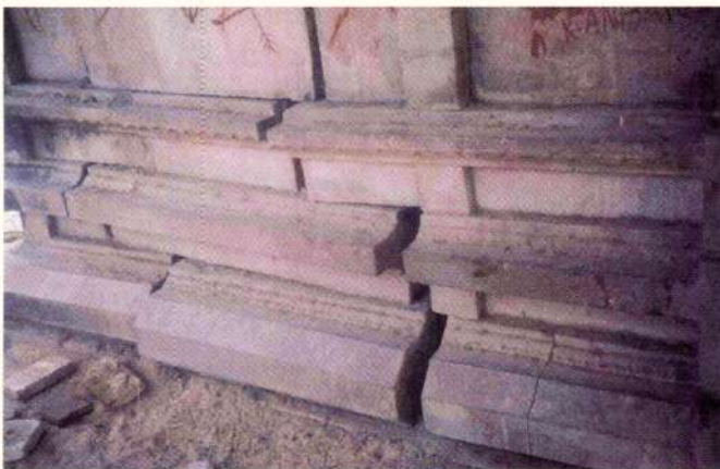
Damaged Upa Peetah
