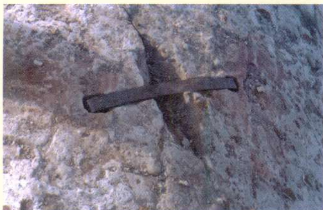
Crack mending method with Copper plate
