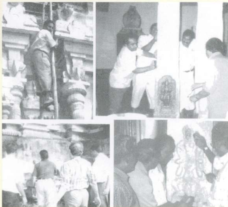
Manual cleaning with liquid Ammonia - the right method of cleaning demonstrated at Meenakshi Sundareswarar Temple, Madurai .
