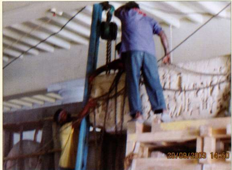
Mounting the suci in the railing
