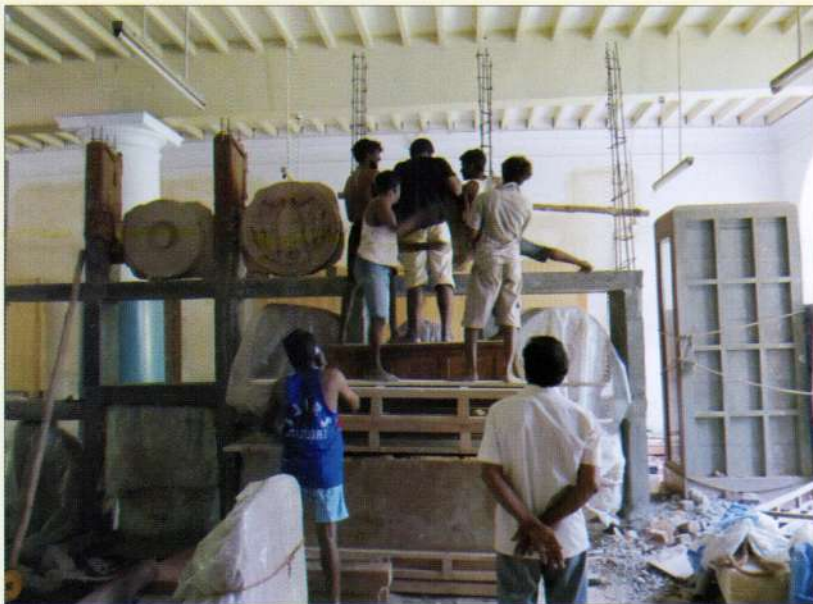
Mounting the suci in the railing
