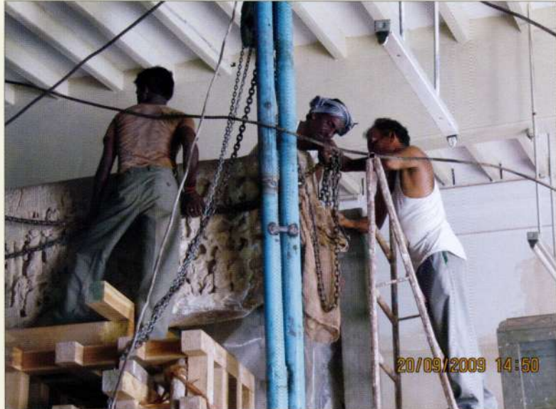
Mounting the suci in the railing
